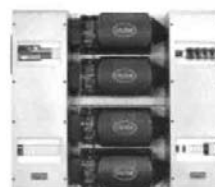
Backup System Outback 9kVA/24 V
